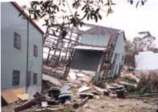
Figure 10. Many structures were destroyed or damaged not only from the strong shaking, but also due to significant fault rupture.
