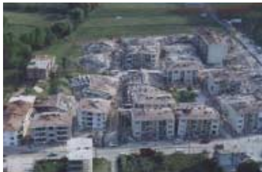
Figure 1. Concrete building collapses in Gölcük after the August 17 th Kocaeli Earthquake in Turkey.
