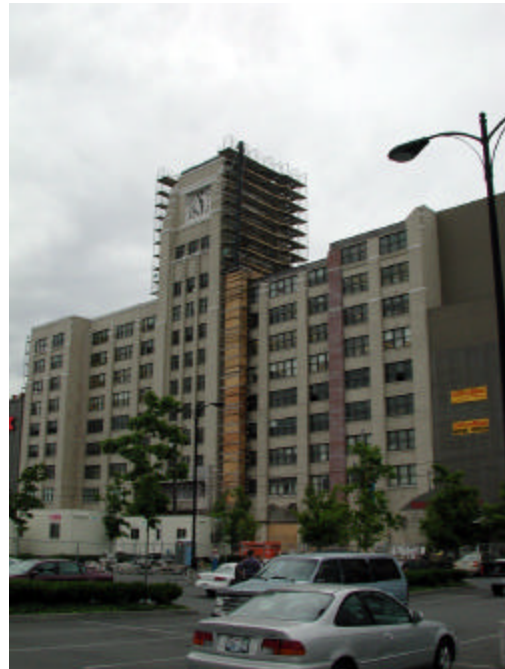
Figure 4 Starbuck's Corporate Headquarters Under Repair, Seattle, WA
