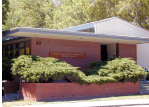
Figure 3 Entrance to the PEER Center
