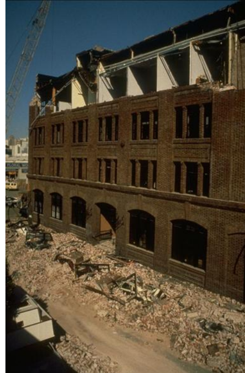
Collapse of inadequately retrofitted brick building onto cars in San Francisco after the 1989 Loma Prieta earthquake.
